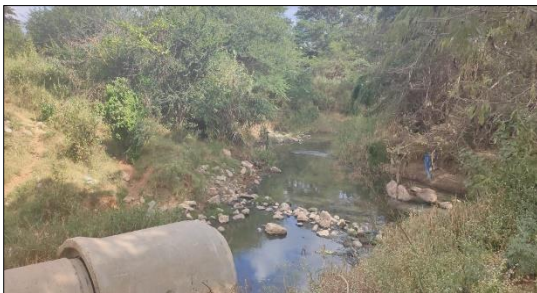
View of the drain inside subject property
